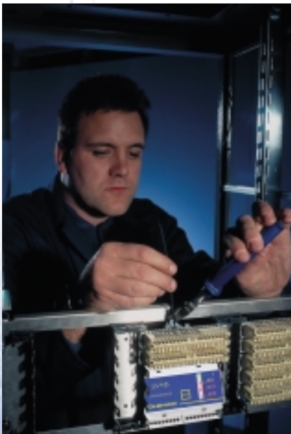
Installation in electric equipment cabinet
